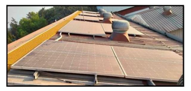
The project activity involves "Solar PV system" as the technology. The system is designed for a capacity of 650 KWp. The solar modules are mounted on module mounting structures of Al-Zn alloy coated steel on top of sheet roofs of the Berger paints manufacturing facility at Rishra.
